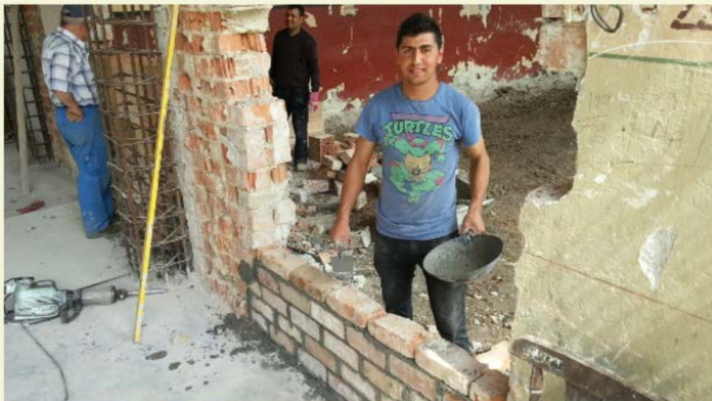
Work continues steadily on the new Vocational Centre in Sacele!
